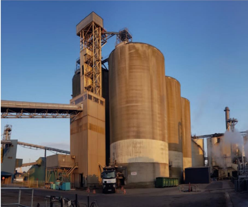
Fig. 1 The Bunge plant in the Port of Brest
