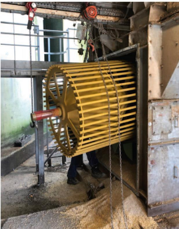
Fig. 3a and 3b The cage pulley is hoisted into the installation
